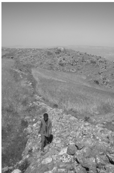
Picture 3 – Wechecha Range: Outer Wall (to the south)
