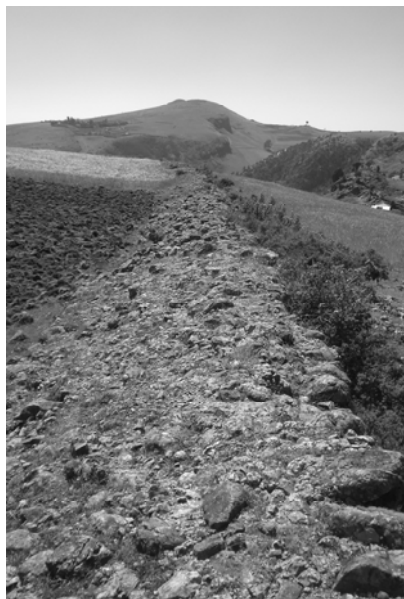
Picture 2 – Wechecha Range: The massive Section Wall to the north
