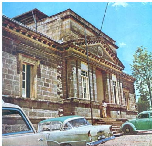
Figure 3.9 Bank of Abyssinia
