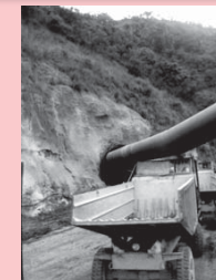
Building an Ethiopian hydroelectric power plant
