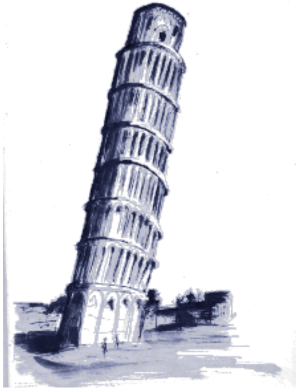
Leaning Tower of Pisa
