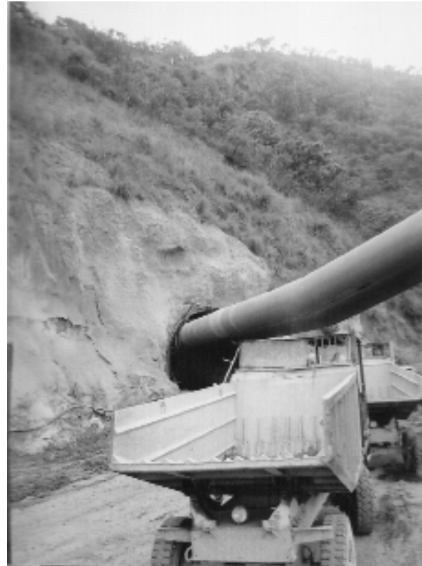
Building an Ethiopian hydroelectric power plant
