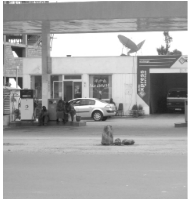
A fuel station
