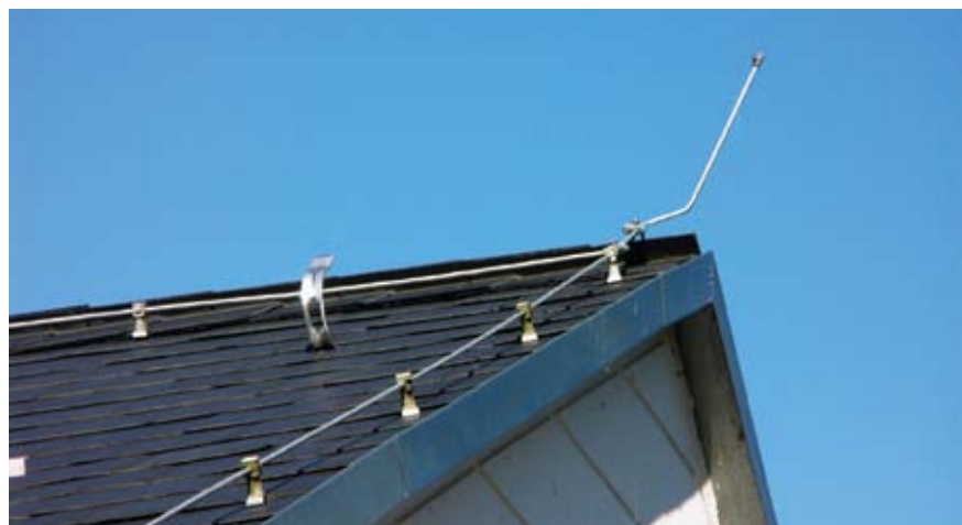
Figure 2.16 A lightning conductor will conduct electric charge from lightning safely away from a building to the earth.
